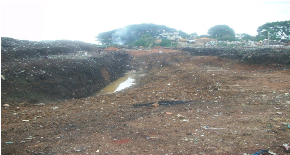
Photo – Foundation footing for Construction of Garage cum workshop
