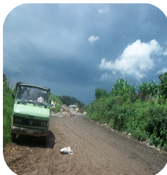
Photo 2: The present condition of access road to the landfill construction site
