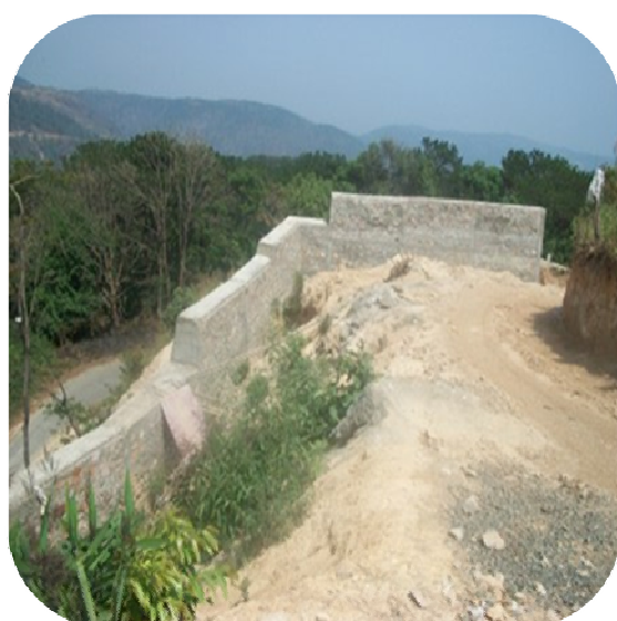
Photo 1: Retaining wall under construction at Sanitary Landfill Site in Marten, Mawiong
